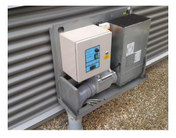
This site now benefits from the protection of a clean air blanket. Two externally wall mounted Positive Pressurisation deliver clean fresh air below the building. The system out performs traditional passive solutions dilute to and disperse accumulating ground gas to create and maintain a Clean Air Blanket system of gas protection.
